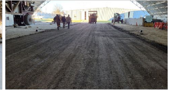
(b) Test section during initial compaction
