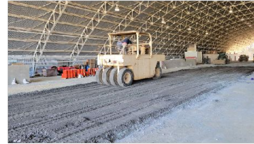
(a) Initial compaction with pneumatic tire roller
