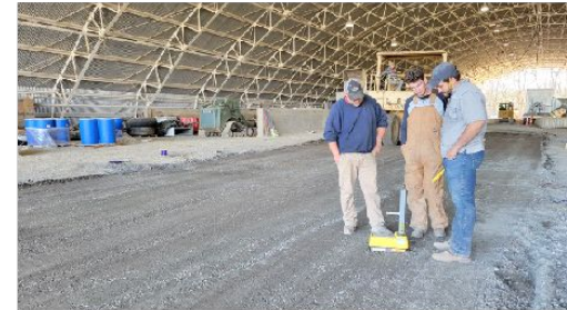
(c) Field density testing during compaction
