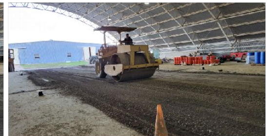
(f) Final compaction with steel drum roller
